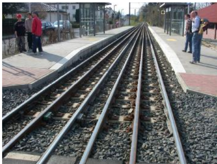
Figure 2: Kassel's solution to solve free profile issues in stations (source: EPFL-LITEP)
