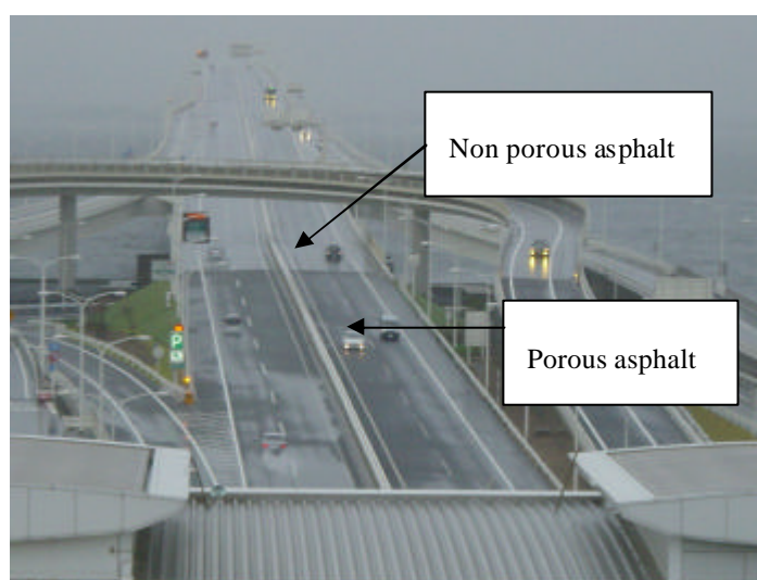
Figure 1 Aqua line crossing Tokyo Bay during a rain storm
